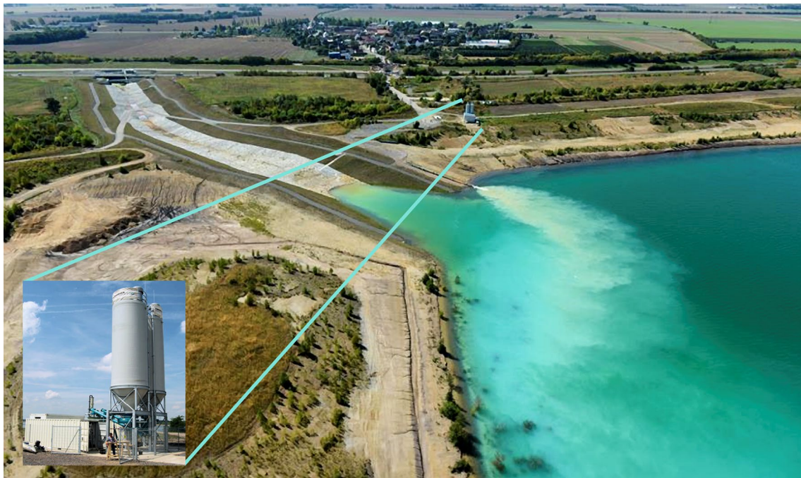
Fig. 8 Stationary neutralization plant on Lake Zwenkau and the lime plume spreading into the water body (image provided by LMBV)
